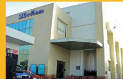
Solar Panel Plant, Baddi (Himachal Pradesh)
