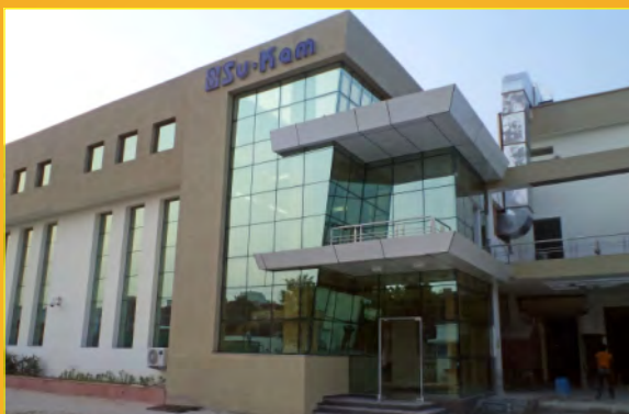
Tubular Battery Manufacturing Facility at Baddi
