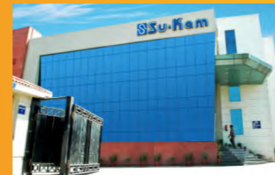
Inverter Plant, Baddi (Himachal Pradesh)
