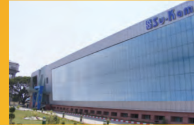
Battery Plant, Katha (Himachal Pradesh)
