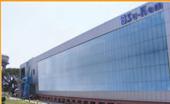
Battery Manufacturing Facility at Katha, Baddi
