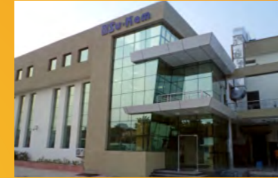
Battery Plant, Baddi (Himachal Pradesh)
