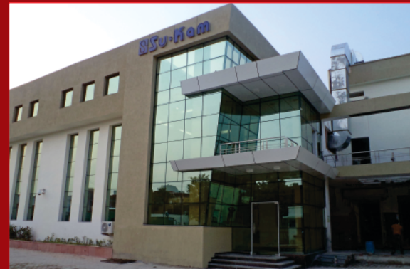
Tubular Battery Manufacturing Facility at Baddi
