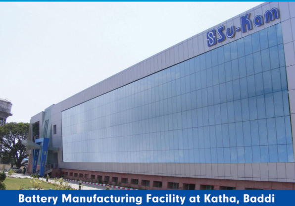
Battery Manufacturing Facility at Katha, Baddi
